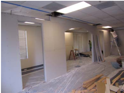
Our New Icon Screen being constructed
